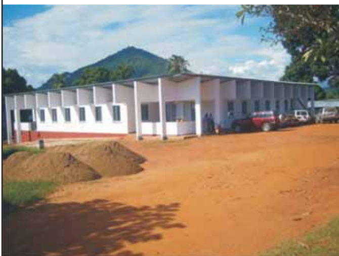
Newly constructed and well equipped Korogwe Laboratory in Tanzania
